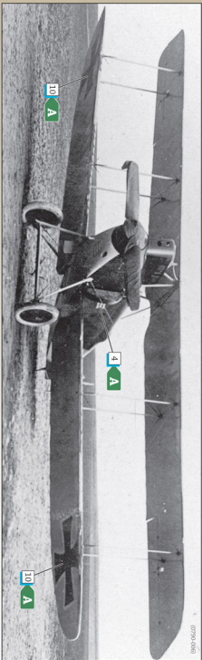
An unidentified mid production LVG built DFW C.V. E fired with its winter cowling. Note the canvas propeller cover, open inspection hatches under the wing and LVG factory position of the bottom wing elements with white outlines.
