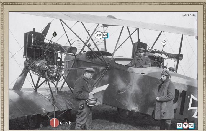
Only the additional angle of incidence markings on the bottom wing and wide gap starting near the trailing edge help identify this as an AEG G.IVb (we have not noted these details on any confirmed AEG G.IV images). Note the different coloured lagging wrapped around each carburetter intake pipe, 3 colour camouflage and the number 21 painted on the fuselage.
