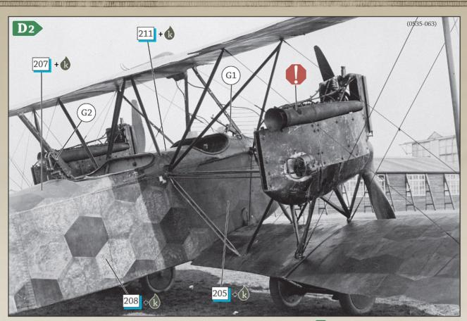
Rear view of the starboard engine nacelle and fuselage from captured AEG G.IV 1125/16 D. Note the uncommon mix of LMG 14 (G2) and LMG 14/15 (G1) Parabellum machine guns for the front and rear armament.
