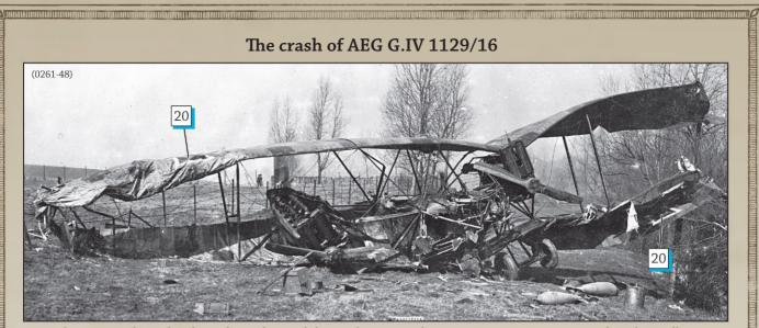
Internal stowage and PuW bombs are littered around the wreckage. Note the uncommon counter rotating Behrend propellers.
