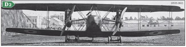
Front view showing the replacement port propeller. AEG G.IV 1125/16 is one of the few aircraft fitted with counter rotating propellers as shown in this photo.
