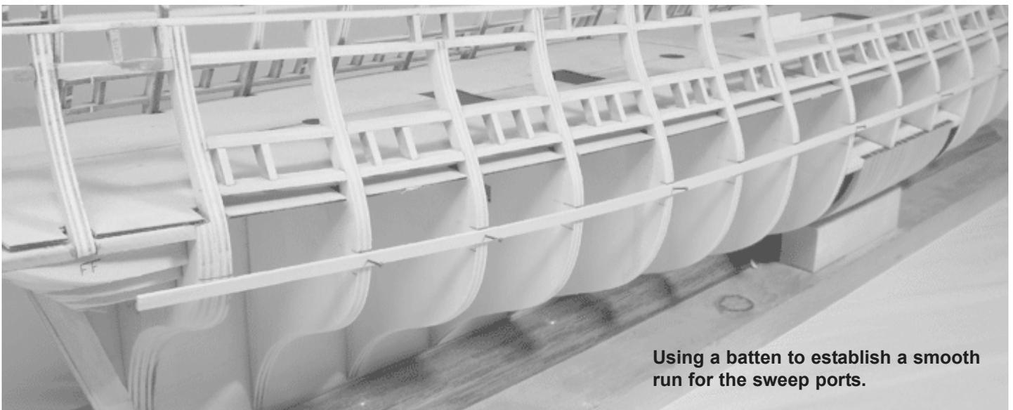
**Using a batten to establish a smooth run for the sweep ports.**
