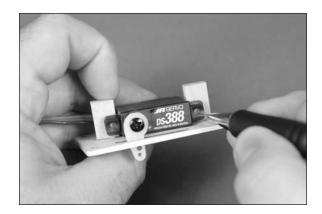
□□ 14. Use a drill and 5/64-inch (2mm) drill bit to drill the holes for the mounting screws. Use care not to enlarge the holes any larger than the drill bit.
