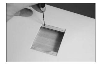
$\Box$  20. Use a #1 Phillips screwdriver to run a 2mm x 8mm self-tapping screw in each of the holes to cut threads in the surrounding wood. Remove the screw before proceeding to the next step.
