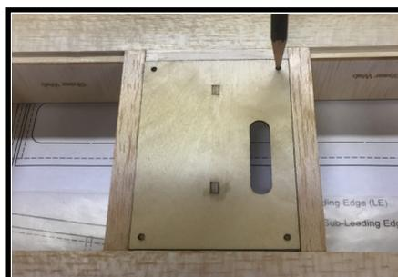
54. Use the hatches as guides to mark the locations of the hatch retaining screws. Drill pilot holes for the screws using a .050" – 1/16" bit.
