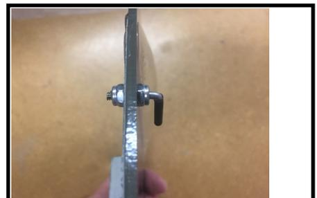
31. Install the handles onto the doors, facing forward.
