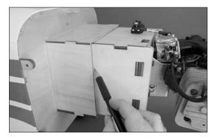
□ 14. Use 30-minute epoxy to secure the engine mounting box in the fuselage. Make sure to apply epoxy to all surfaces that will come in contact with each other on both the engine mounting box and fuselage. Slide the engine mounting box back into position and use isopropyl alcohol and a paper towel to remove any excess epoxy.
