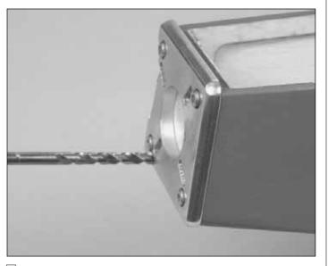
■ 4. Use the hole in the mount as a guide to drill a 3/16" [4.8mm] hole through the firewall. **Note:** It is okay if you drill through a portion of the factory-installed blind nut on the back of the firewall. Remove the mount.
