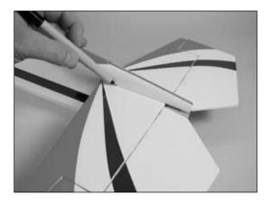
O 6. Use a sharp hobby knife to cut the covering slightly inside the lines drawn. Be very careful not to cut into the underlying wood, as this will weaken the stab and cause it to fail in flight.
