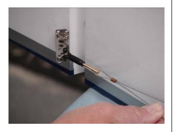
12. Loop the cable back through the brass swage tube as shown.
