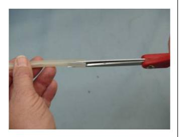
20. After splitting the silicon tubing cut off one side of the split section as shown. This will provide a relief section of the tubing for the nylon tie lock and insulate it from the metal pipe surface.
