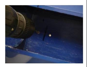
6. Locate the two plywood canister mounting doublers with pre-installed blind nuts as shown.
